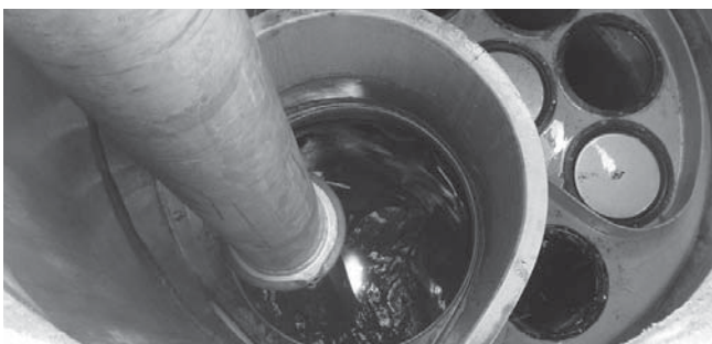
Vacuuming Sump Through MAW
