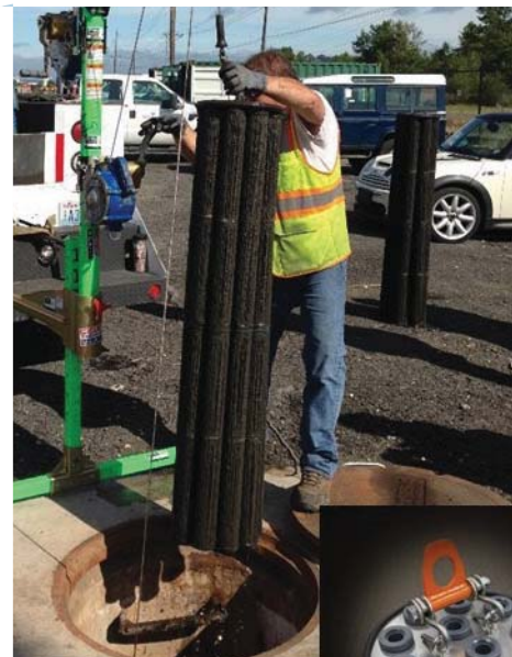
Cartridge Removal & Lifting Device
