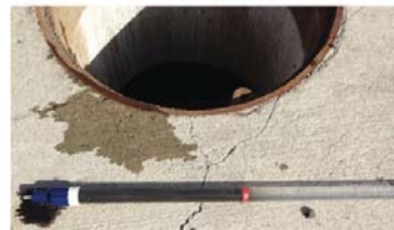
Inspection Utilizing Sediment Probe
