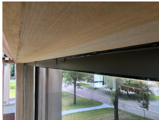
Line 1 CW H-J: Snap on cover cannot be removed. 1. The cedar board of the horizontal soffit butts to the top face of the aluminum curtainwall frame @ the north side jamb. 2. The cedar board butts +/- 1/4" below the top of the aluminum curtainwall frame at the far south side jamb. 3. There is no head joint/reveal for the primary sealant. The cedar board butts directly to aluminum curtainwall frame and the sealant/residue is only left on the aluminum curtainwall frame.
