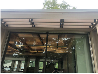
Line 1 CW F-G: cover/sealant removed
