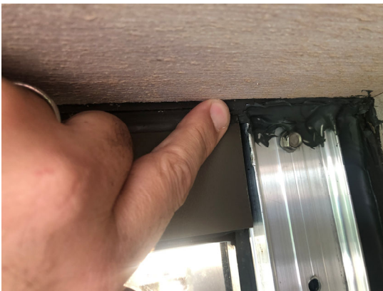
Line 1 CW H-J: Snap on cover cannot be removed. 1. The cedar board of the horizontal soffit butts to the top face of the aluminum curtainwall frame @ the north side jamb. 2. The cedar board butts +/- 1/4" below the top of the aluminum curtainwall frame at the far south side jamb. 3. There is no head joint/reveal for the primary sealant. The cedar board butts directly to aluminum curtainwall frame and the sealant/residue is only left on the aluminum curtainwall frame.
