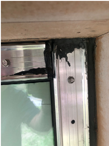
Line 1 CW F-G: (+/-)1/4" max exist joint
