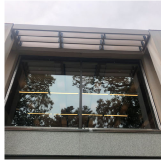
Line 1 CW H-J & K-L: covers/sealant NOT removed @ heads
