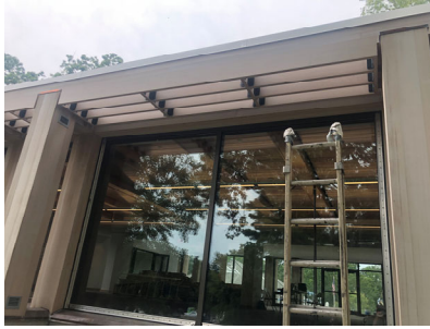
Line 1 CW H-J & K-L: covers/sealant NOT removed @ heads
