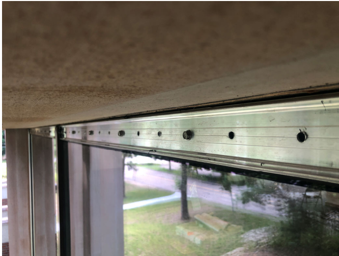
Line 1 CW F-G: Primary sealant cannot be installed - exist joint @ (+/-) 1/4" to 0"
