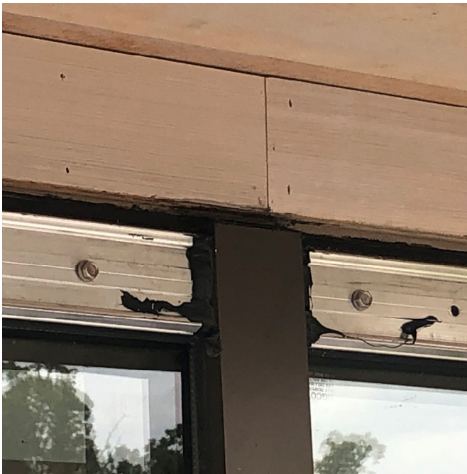
Line 6.9 CW F-G & K-L: Finished cedar board at bulkhead to align with face of aluminum curtainwall frame.
