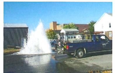
Backsiphonage may occur due to a water main break or other low-pressure incident such as a fire.
