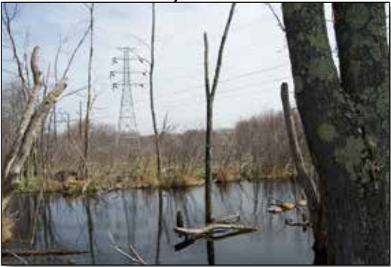
PHOTO 2.1: Large transmission lines are near these sensitive wetlands, which leads to concerns about the potential impact of utility maintenance regimes on the water quality.
